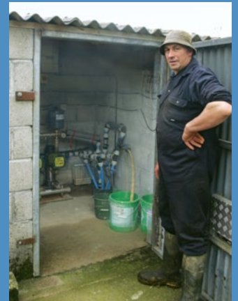
The farm's old electric pump and filter system.
