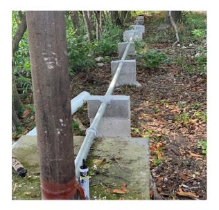
When the supply pipe is above ground it will need anchoring, this can be done with concrete blocks like you can see in the picture to the left.
